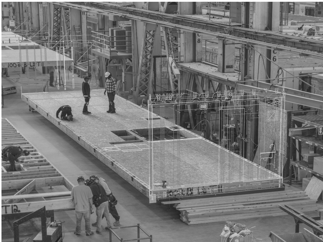
Modular housing production floor with BIM overlay showing framing
